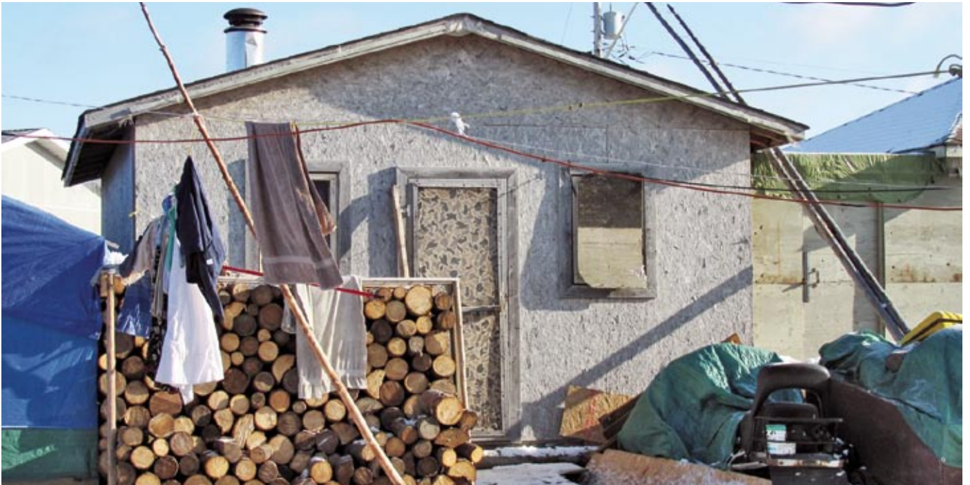
Due to the shortage of houses in the Attawapiskat First Nation community, shacks like this are being used as homes.
