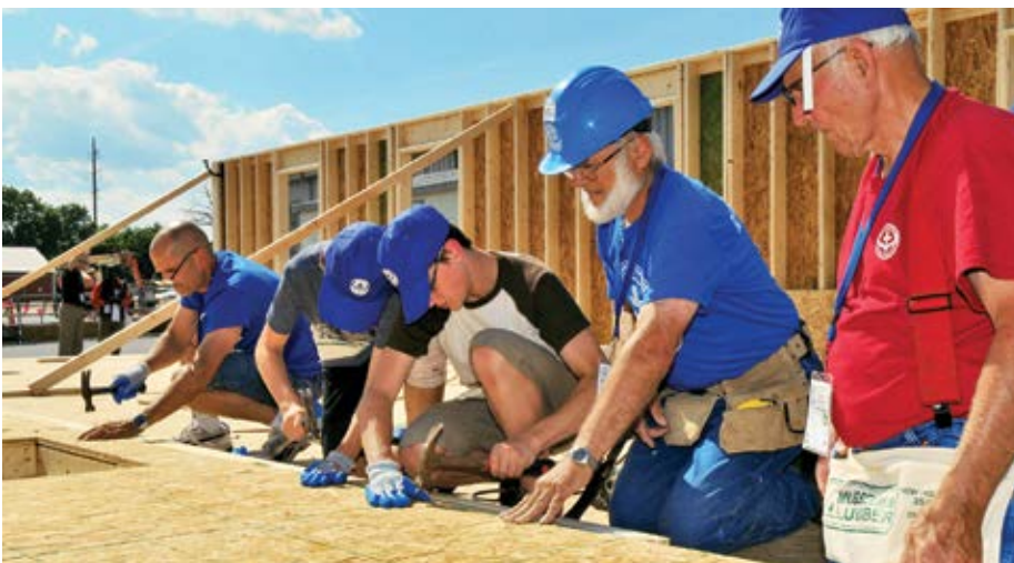
Two prefabricated houses were built for Mennonite Disaster Service at PA 2015. MDS staff were on hand every afternoon to guide volunteers in constructing the floors and walls for houses destined for two families who lost their homes in natural disasters, one in Nebraska and the other in Maryland.
