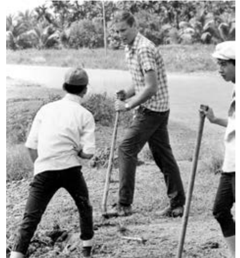
In 1967 Gary Dewarle of Saskatoon (in the checked shirt) helped to build a road at a refugee camp near Saigon, South Vietnam.
