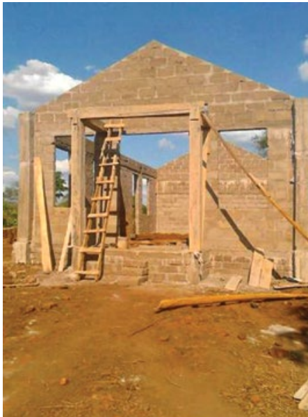
A new church building for Msikisi, Tanzania, is under construction.
