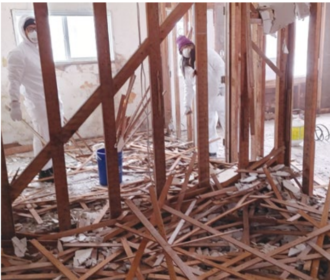
Stephanie Ho and Ray Tsan were involved in some serious demolition.
